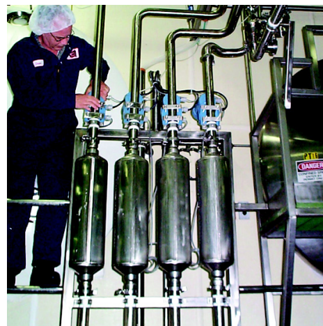
Direct mass measurement of products flowing through Micro Motion 3A authorized T-Series meters has helped to improve first-pass yields at Perry's by 15%
